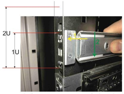
Do so with all 4 Mount Points. You can fix the Rail with the screws outside the Rail.
